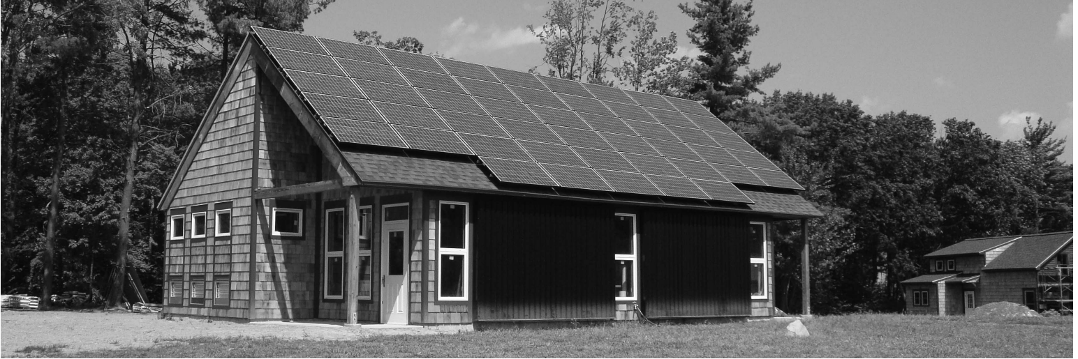
At Noble View Outdoor Center, the bathhouse's exterior is completed. It's expected to be open this November. photo by Gary Forish
